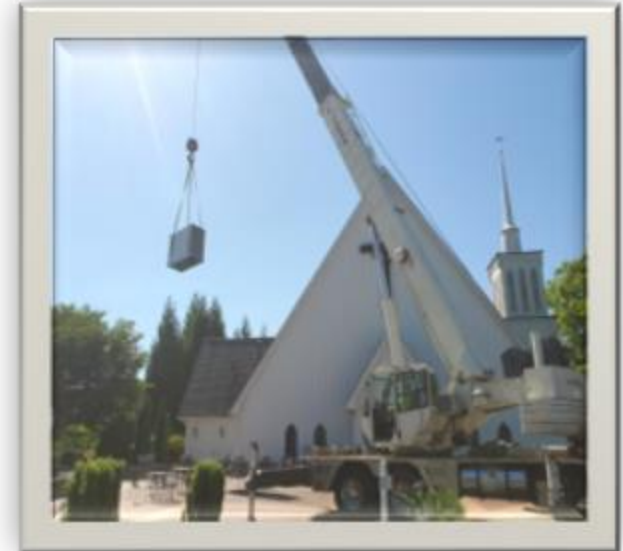
Replacement of Air Conditioning Unit
